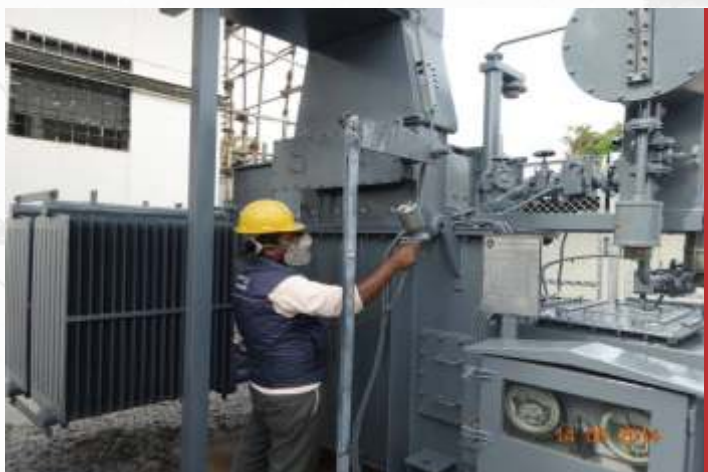
Painting at site
